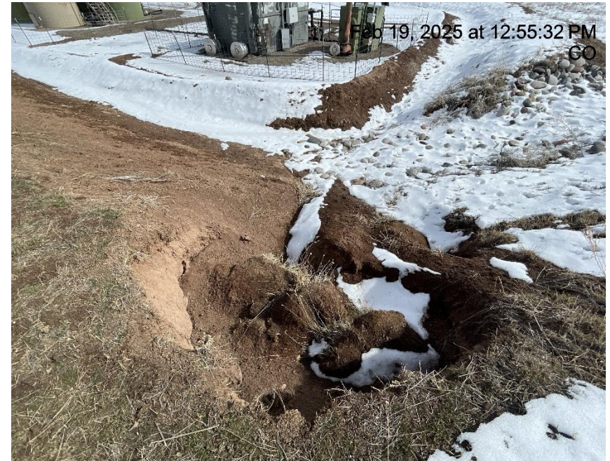
Photo # 7210 Lack of stabilization/sloughing/wildlife hazard
