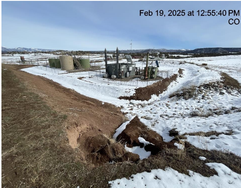
Photo # 7209 Lack of stabilization/sloughing/wildlife hazard
