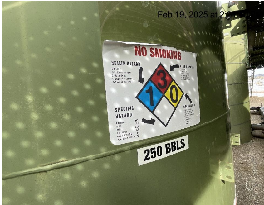
Photo # 7539 Tank label missing required information
