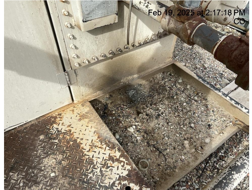
Photo # 7534 Staining near separator
