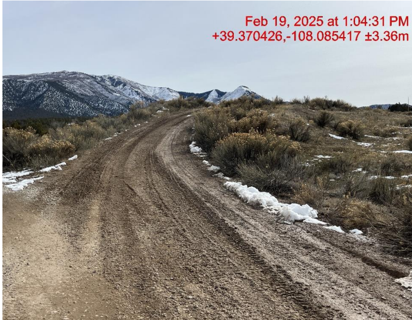
Photo # 5419 Tracking onto lease road/Insufficient tracking BMP's
