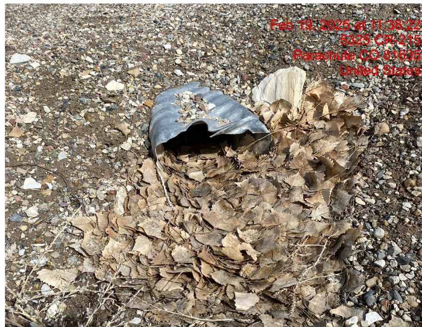
Damaged Culvert – Photo #06728
