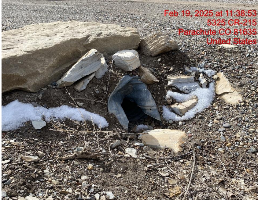
Damaged Culvert – Photo #06729
