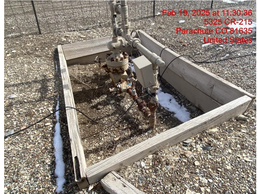
Uncovered Wellhead Cellar – Photo #06723
