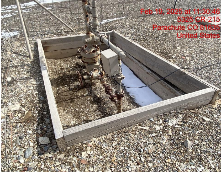
Uncovered Wellhead Cellar – Photo #06724
