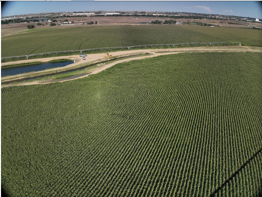
In View – Tank Battery (Loc ID 319013 ), Ditch Road, Flowline EAST – 40.019138/-104.853343
