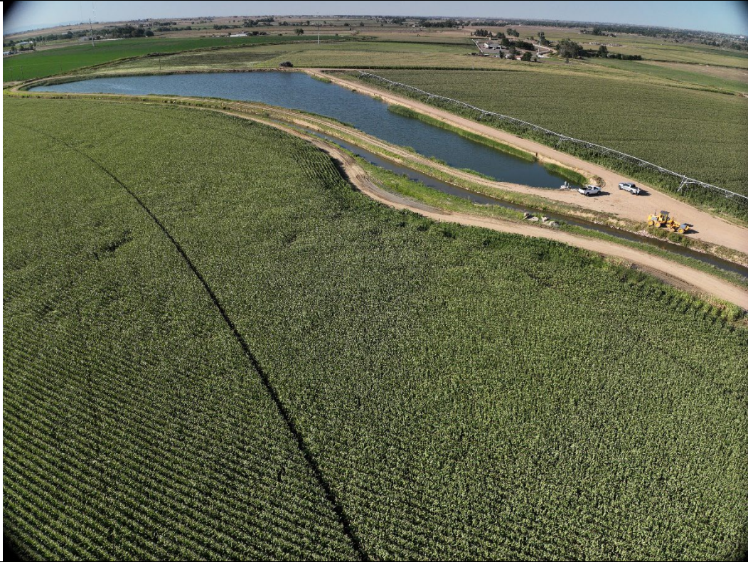
In View – Tank Battery (Loc ID 319013 ), Ditch Road, Flowline NORTH – 40.018444/-104.852183
