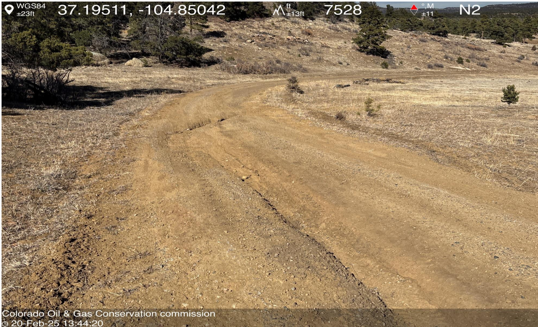
PHOTO 6: STORMWATER BMP'S HAVE FAILED AND CAUSING STORMWATER TO BYPASS CULVERT AND ERODE THE ROW. REPAIR OR INSTALL STORMWATER BMP PER RULE 1002. CA DATE EXTENDED DUE TO WINTER CONDITIONS 4-1-2025.
