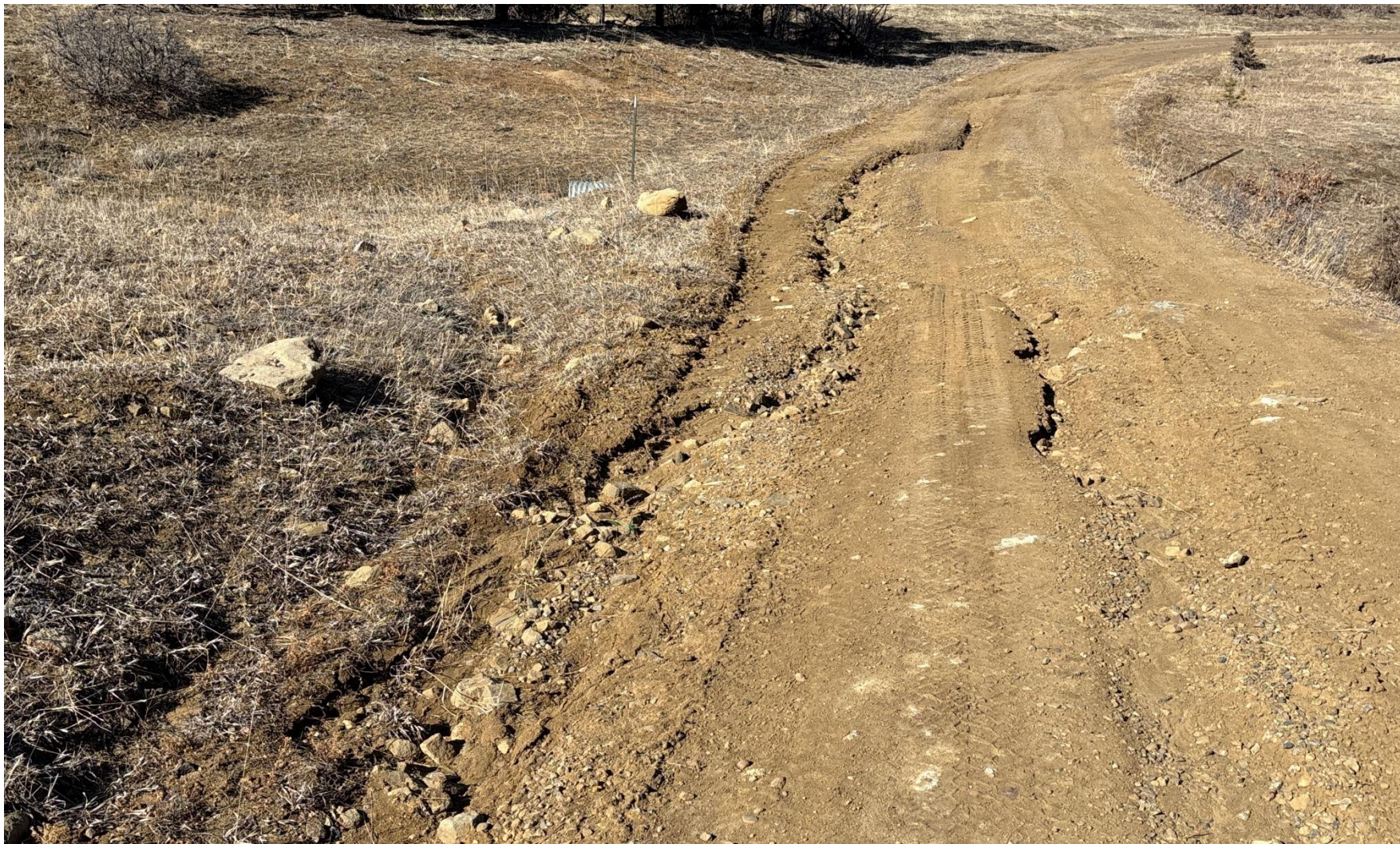
PHOTO 4: STORMWATER BMP'S HAVE FAILED AND CAUSING STORMWATER TO BYPASS CULVERT AND ERODE THE ROW. REPAIR OR INSTALL STORMWATER BMP PER RULE 1002. CA DATE EXTENDED DUE TO WINTER CONDITIONS 4-1-2025.
