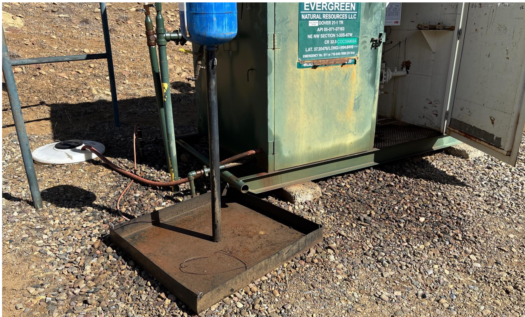
PHOTO 5: AREA OF IMPACTED SOIL NEAR METER HOUSE, Conduct maintenance on equipment, cleanup stained material and review self inspection processes. COMPLY WITH RULE 1002,.(2).D. CA DATE 3-3-2025.
