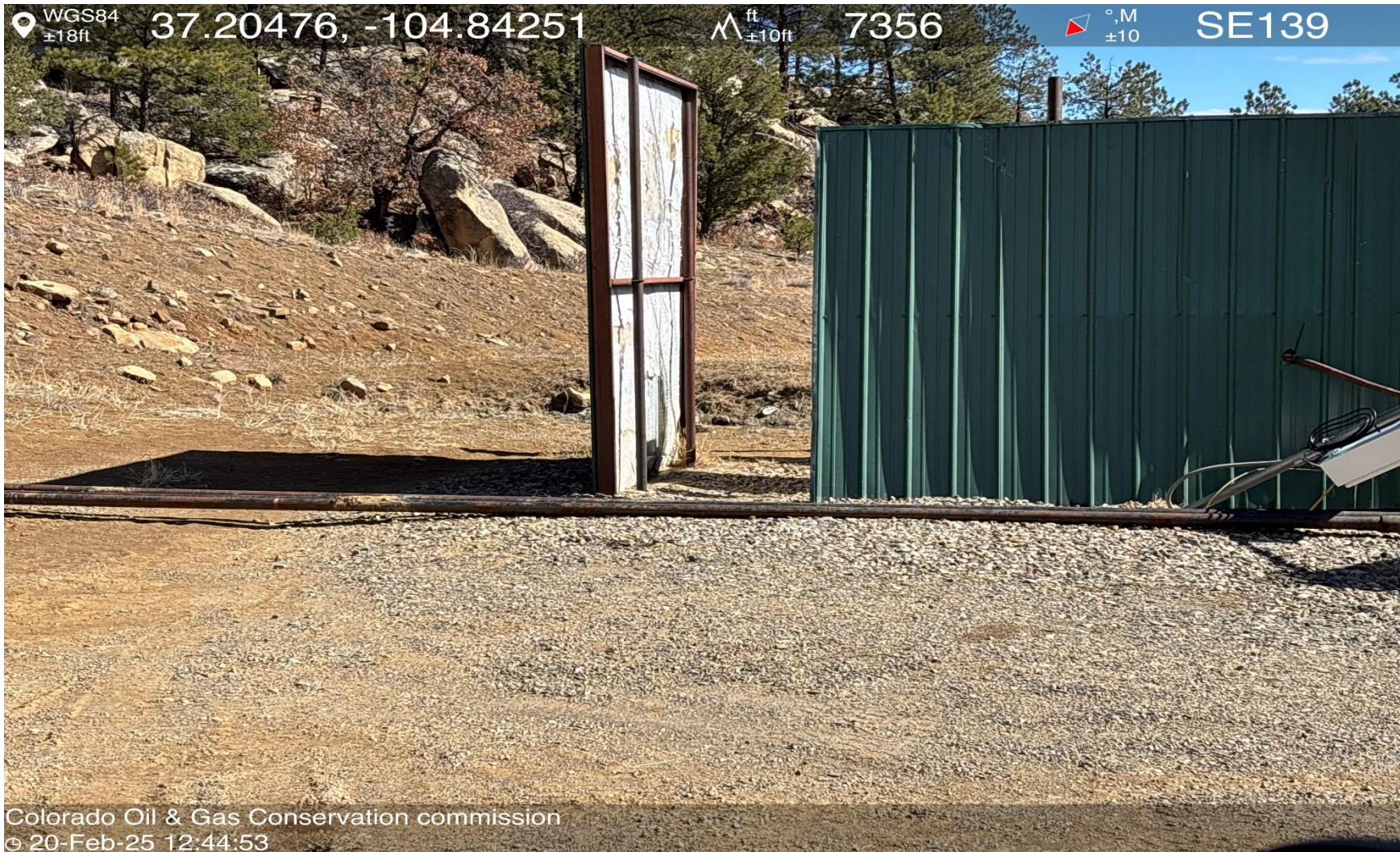
PHOTO 7: UNUSED EQUIPMENT STORED ON LOCATION (TUBING), REMOVE UNUSED EQUIPMENT PER RULE 606. CA DATE 3-3-2025.
