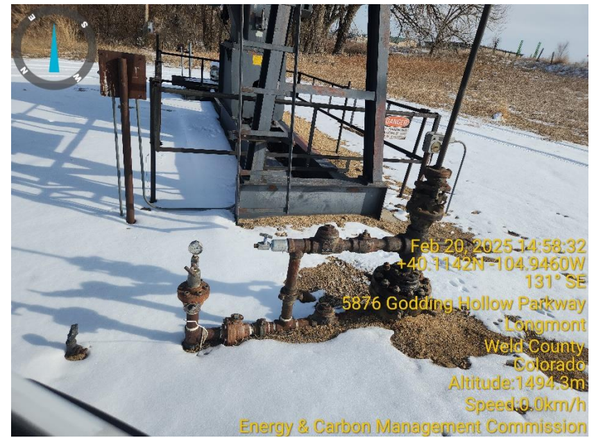
Photo 2 Wellhead Valves open.
