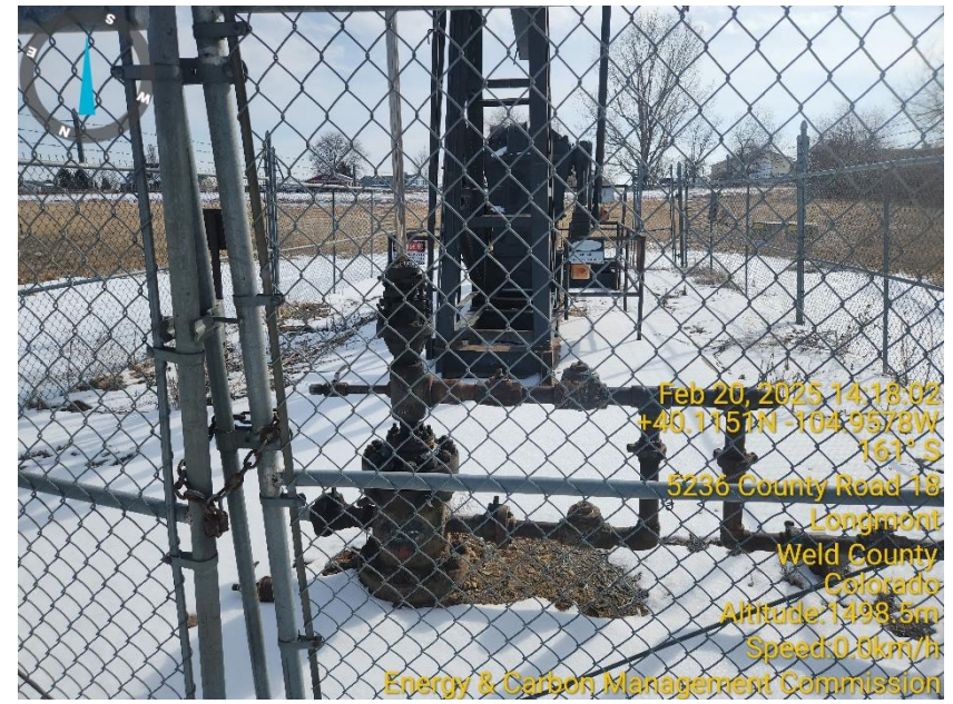
Photo 2 Wellhead Valves open.
