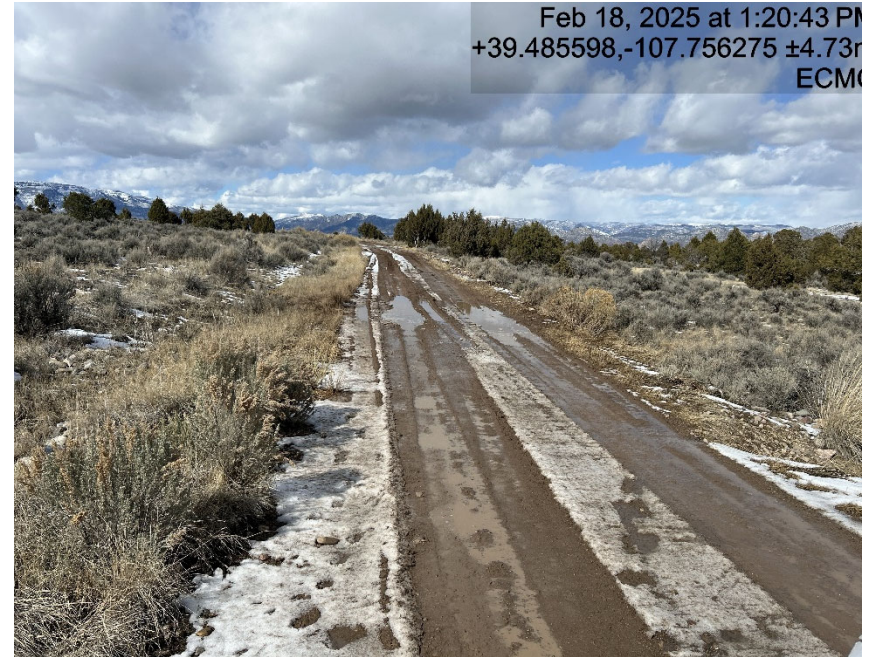
Access road lacks stabilization
