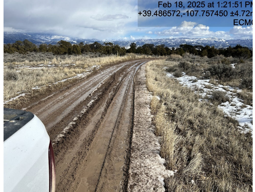
Access road lacks stabilization
