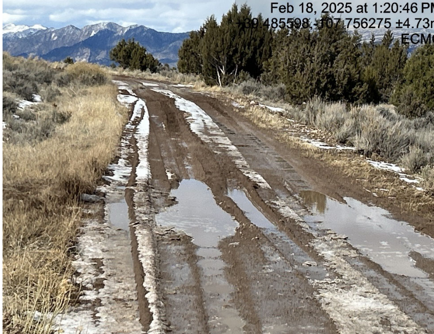
Access road lacks stabilization
