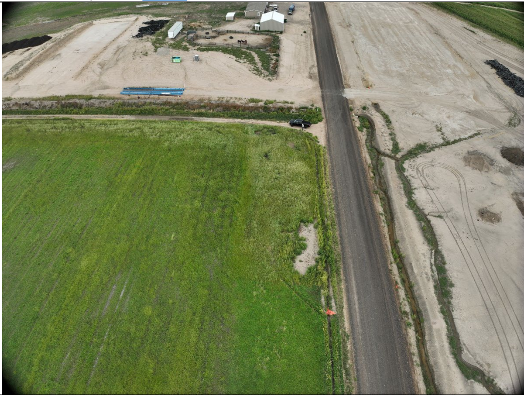
In View – Tank Battery (Loc ID 445077 ), Access Road, Flowline EAST – 40.348851 / -104.479942
