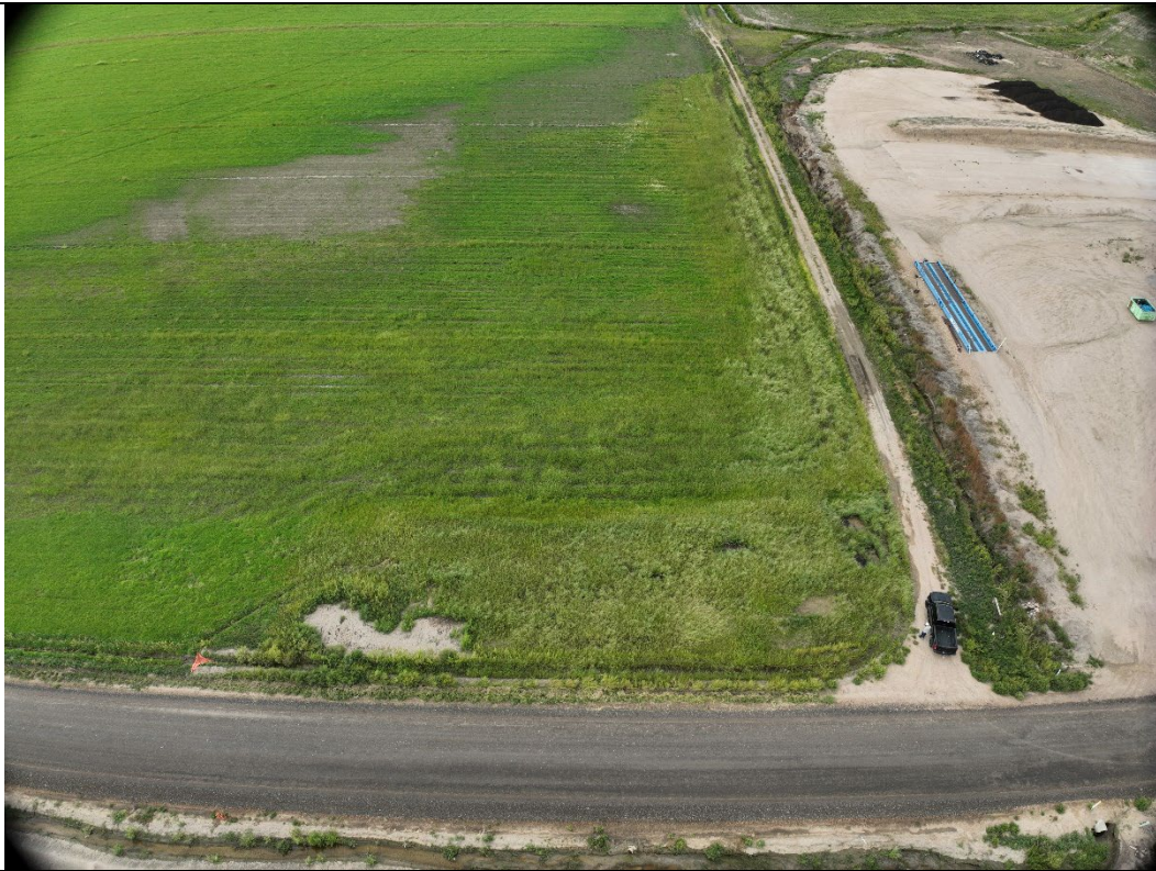
In View – Tank Battery (Loc ID 445077 ), Access Road, Flowline NORTH – 40.348442 / -104.479158
