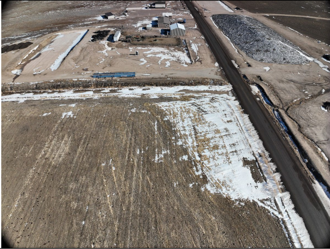
In View – Tank Battery (Loc ID 445077 ), Access Road, Flowline EAST – 40.349051 / -104.479894
