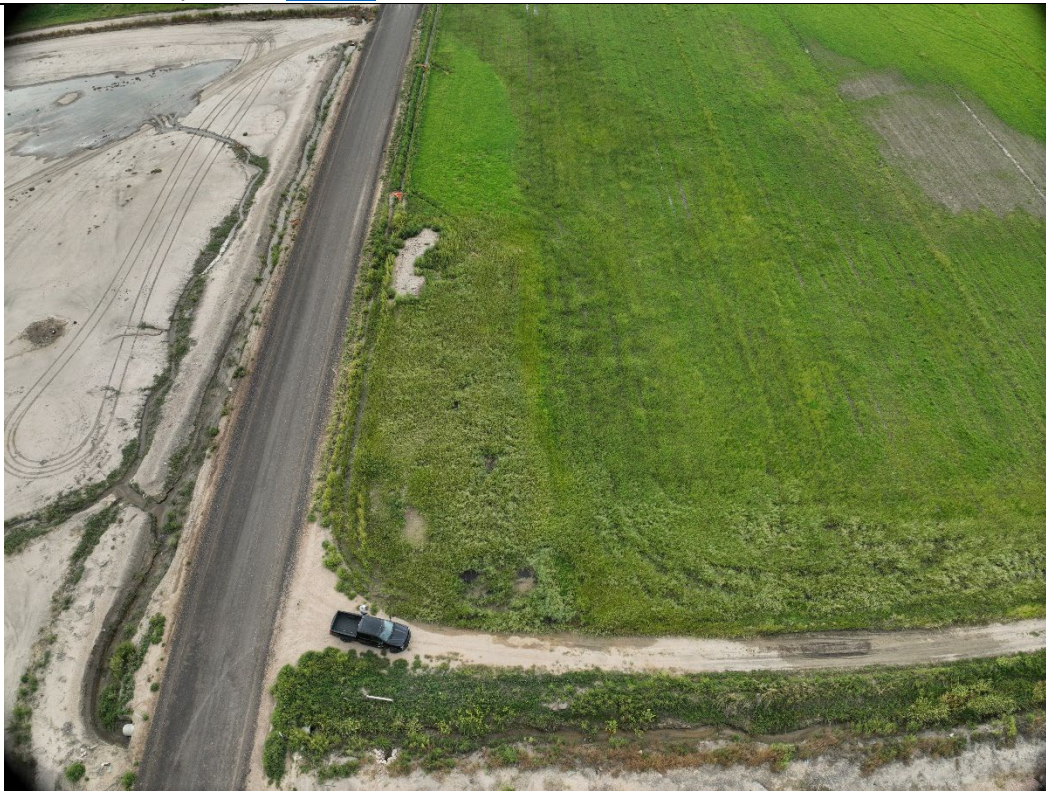
In View – Tank Battery (Loc ID 445077 ), Access Road, Flowline WEST – 40.348914 / -104.478519
