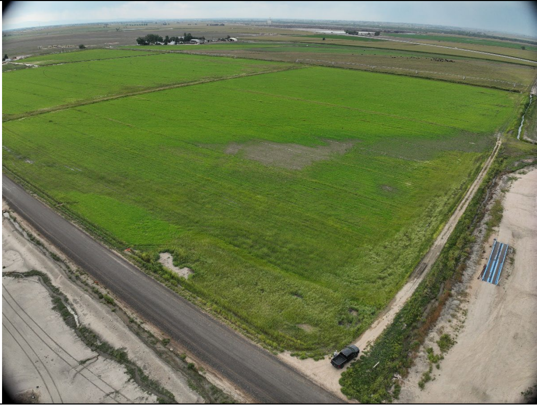
In View – Well, Tank Battery (Loc ID 445077 ), Access Road, Flowline NORTHWEST – 40.348387/-104.478587
