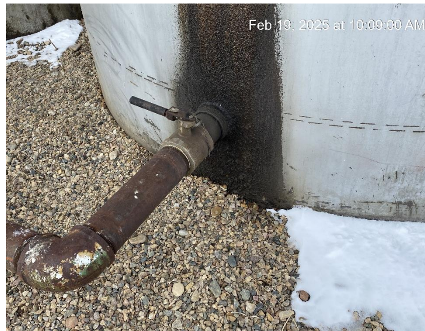
Staining around tanks
