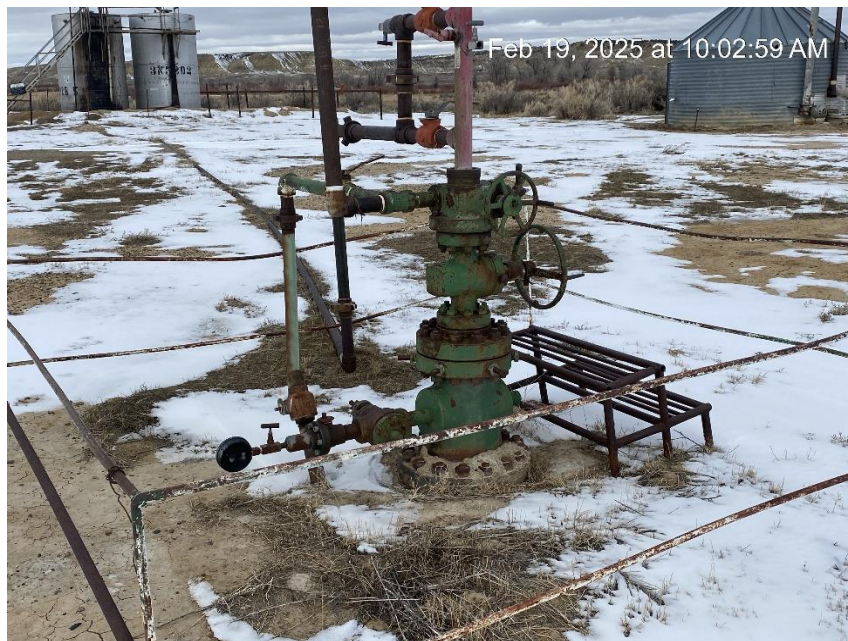
Blow down line to tank missing back pressure valve
