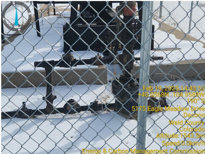
Photo 3 Wellhead valves are shut.
