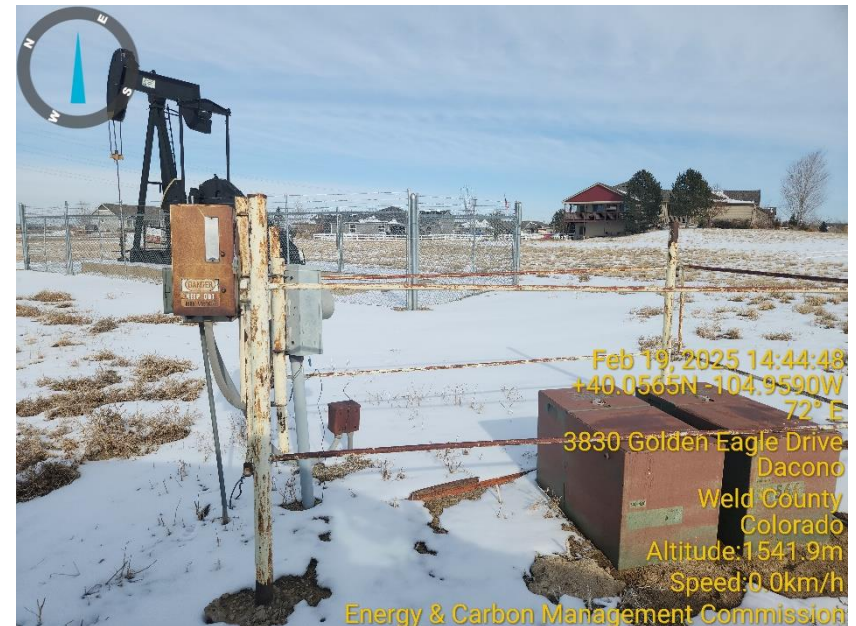
Photo 4 Electric panel & meter box are shut off.
