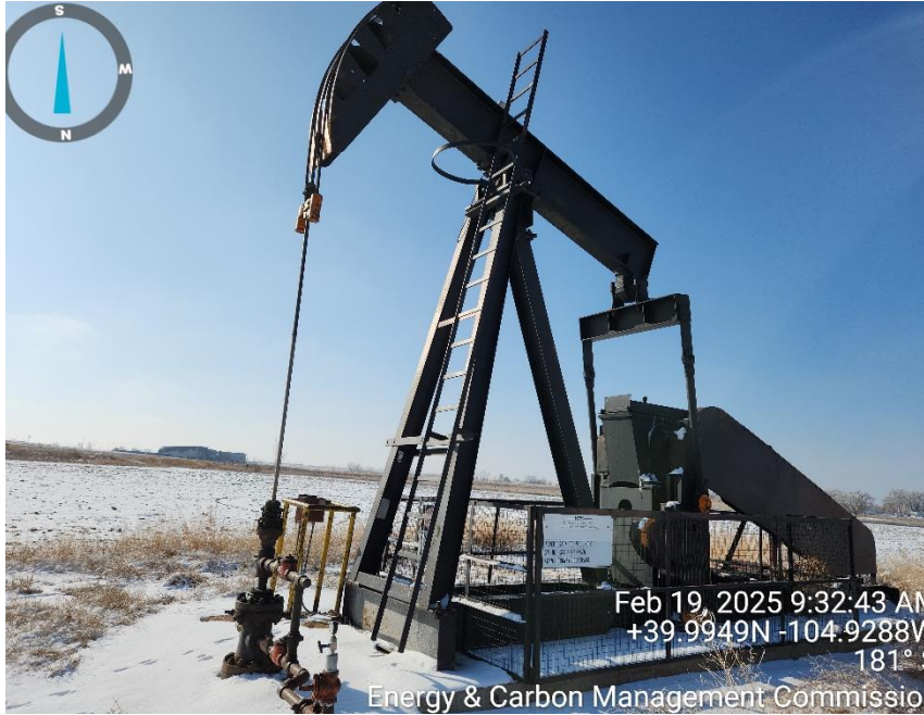
Photo 1 well head and equipment
