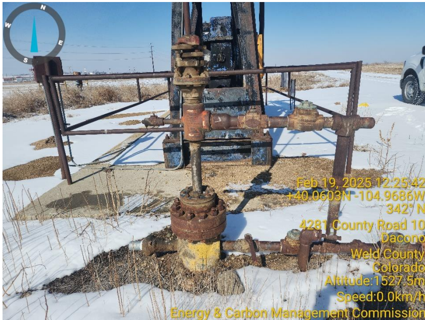
Photo 3 Wellhead valves are closed.
