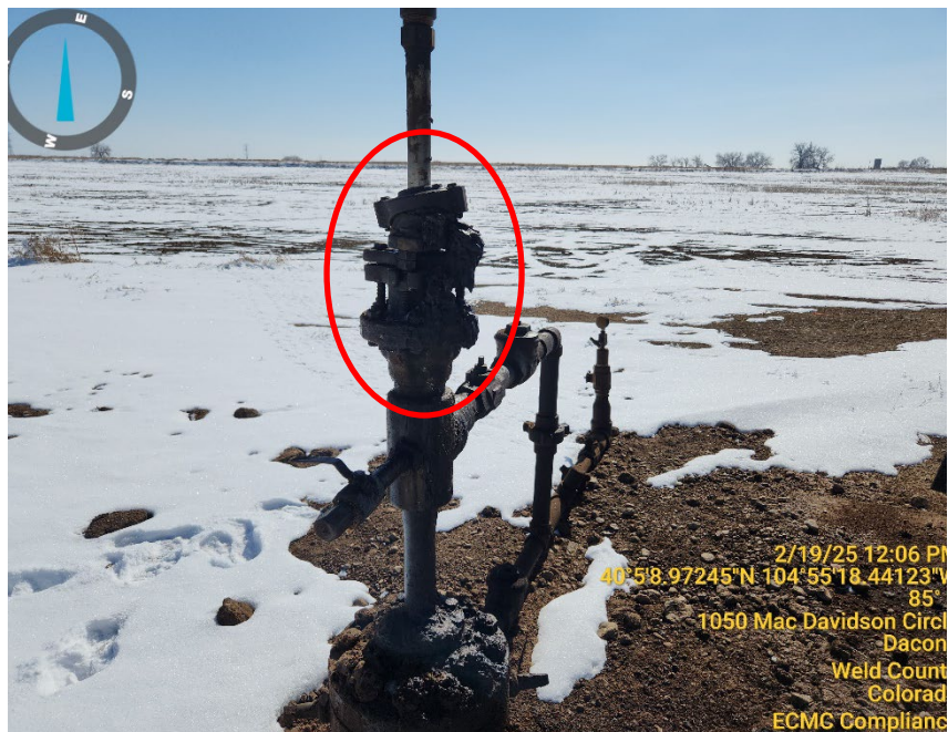
Photo 3: Possible leak, mechanical issue
