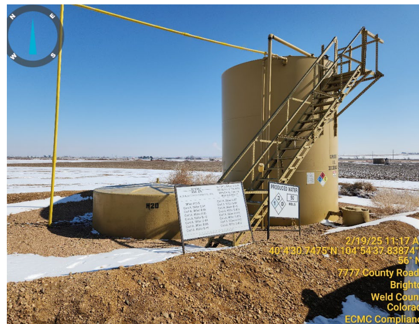
Photo 4: Centralized Tank Battery
