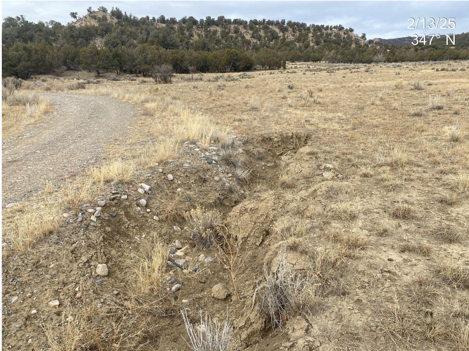
Photo 3. Erosion chanel/pit observed forming at the location access point.
