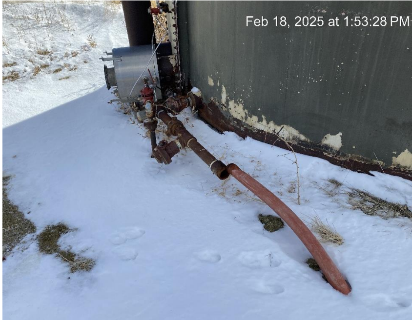
Open end tank valve. Debris.
