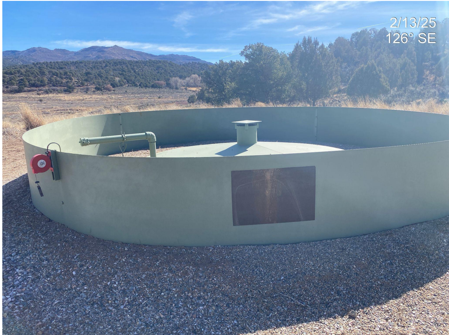
Photo 2. Label at produced water tank is no longer legible.
