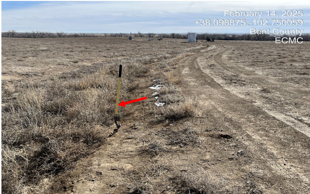
Photo 2. Facing southeast along the access road. There is erosion along the road that must be repaired and stabilized. Red arrow points to 4.5' shovel for scale. Vehicles are driving outside of the original access road to avoid the eroded road.
