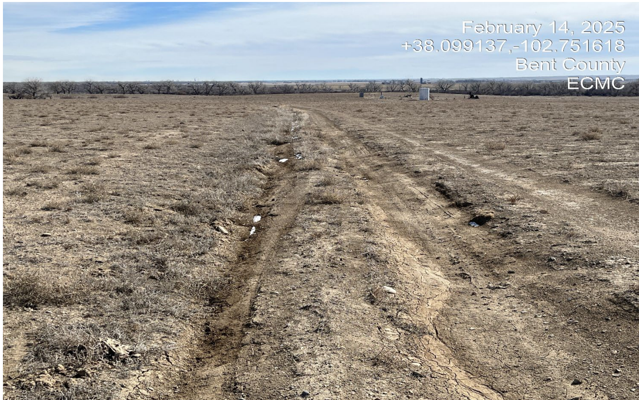
Photo 1. Facing southeast along the access road. There is erosion along the road that must be repaired and stabilized. Vehicles are driving off the original road causing more disturbance.
