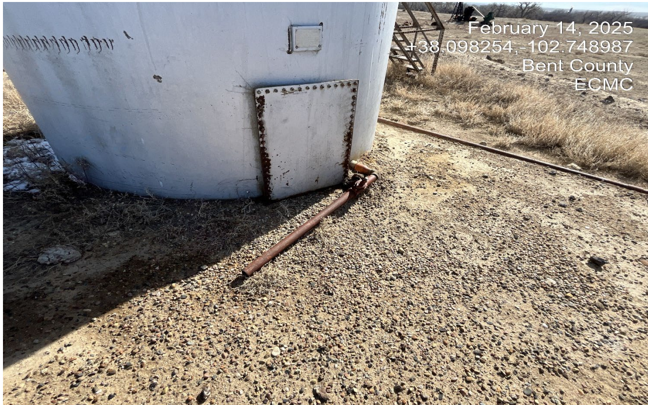
Photo 4. Stained soil have faded but still remain at the base of the tank.
