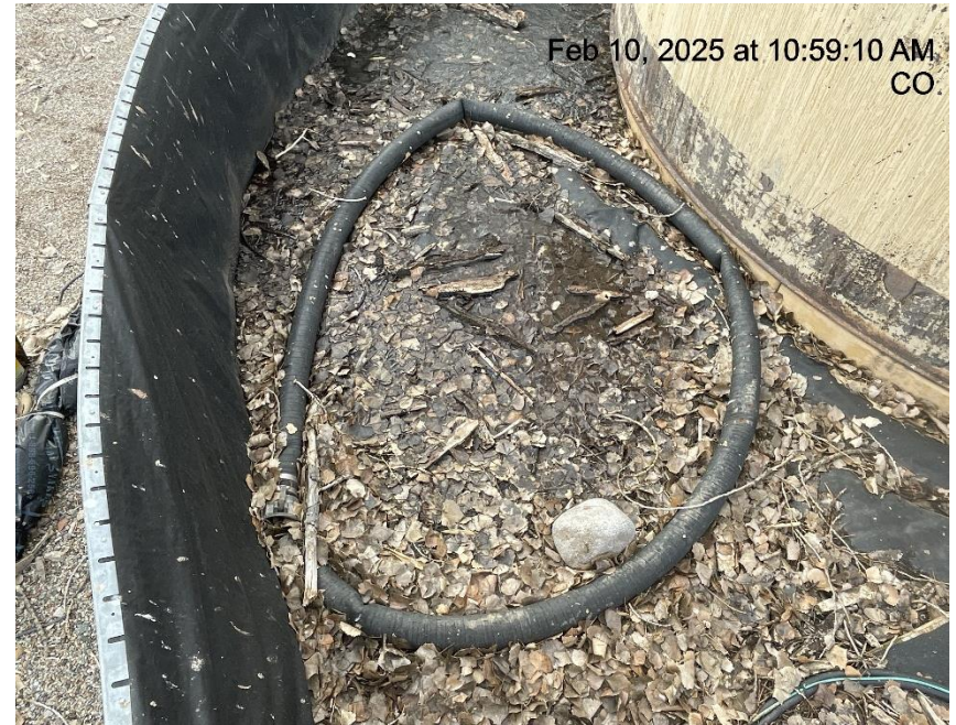
Photo # 4459 Damaged hose/debris
