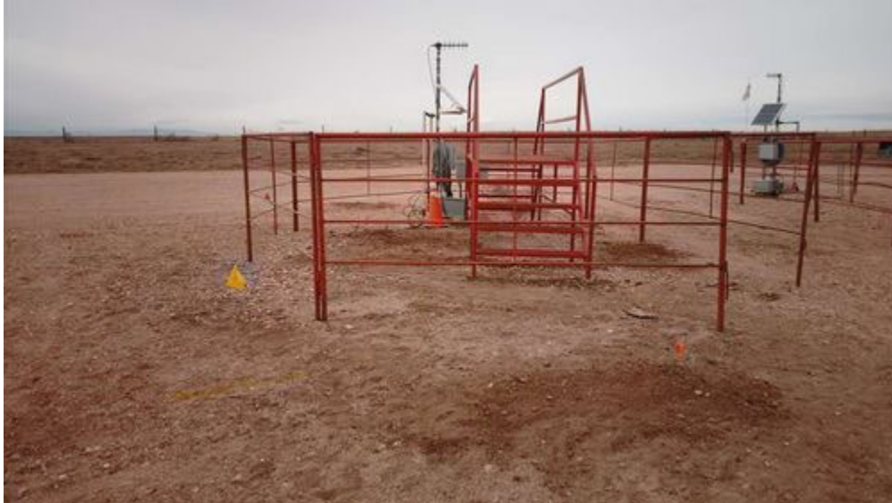
Wellhead Excavation Sampling Closure Photo
