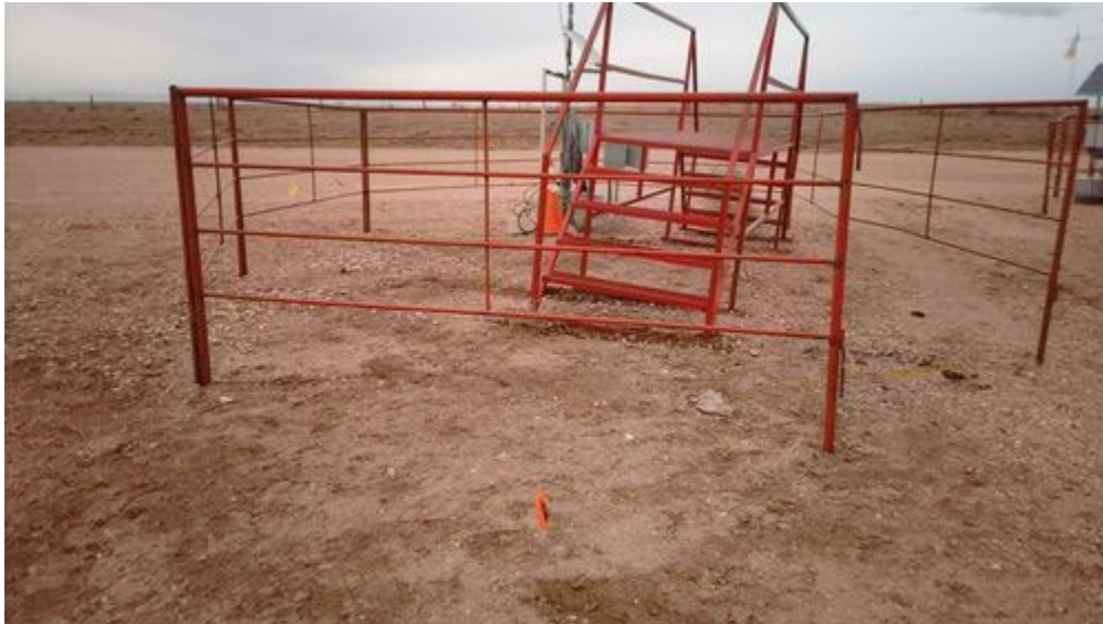
Initial Wellhead Excavation Photo
