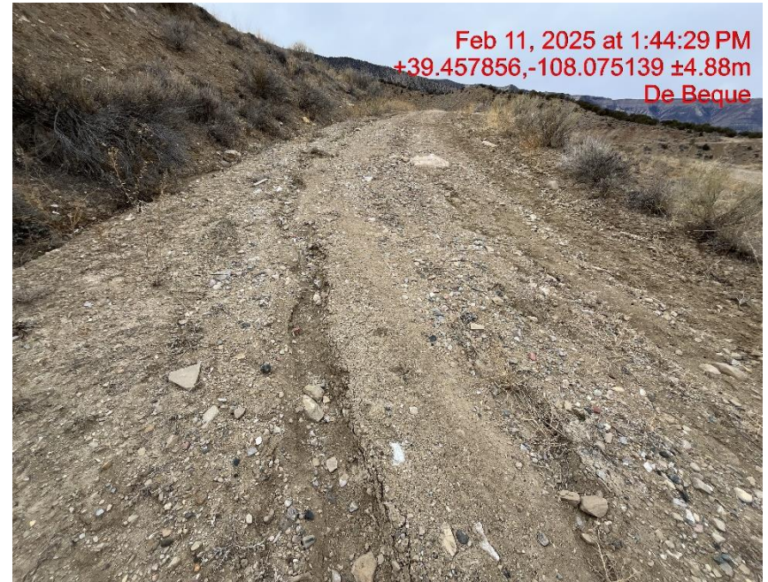
Photo # 4794 Rill erosion on access road, south side of location
