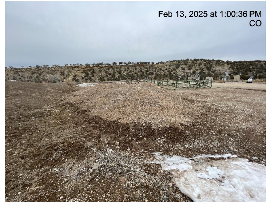
Photo # 5645 Stockpiled soils with no BMP's
