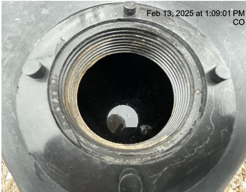
Photo # 5638 Failure to maintain chemical BMP – Chemical tank containment approximately 7/8 full of fluid/BMP insufficient to contain possible spill
