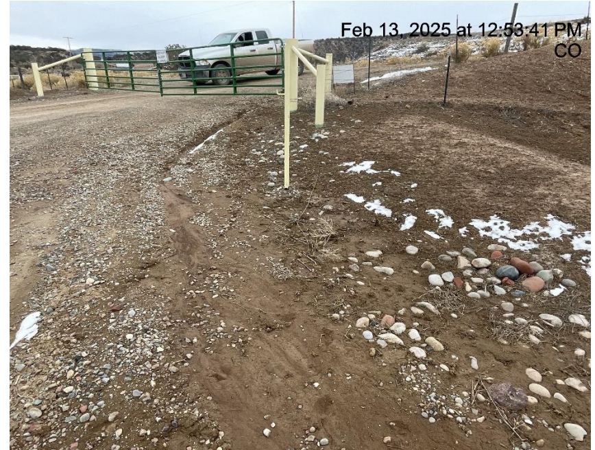
Photo # 5649 Erosion & transport of sediment/insufficient BMP's
