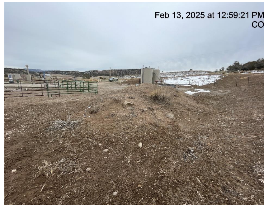
Photo # 5643 Stockpiled soils with no BMP's
