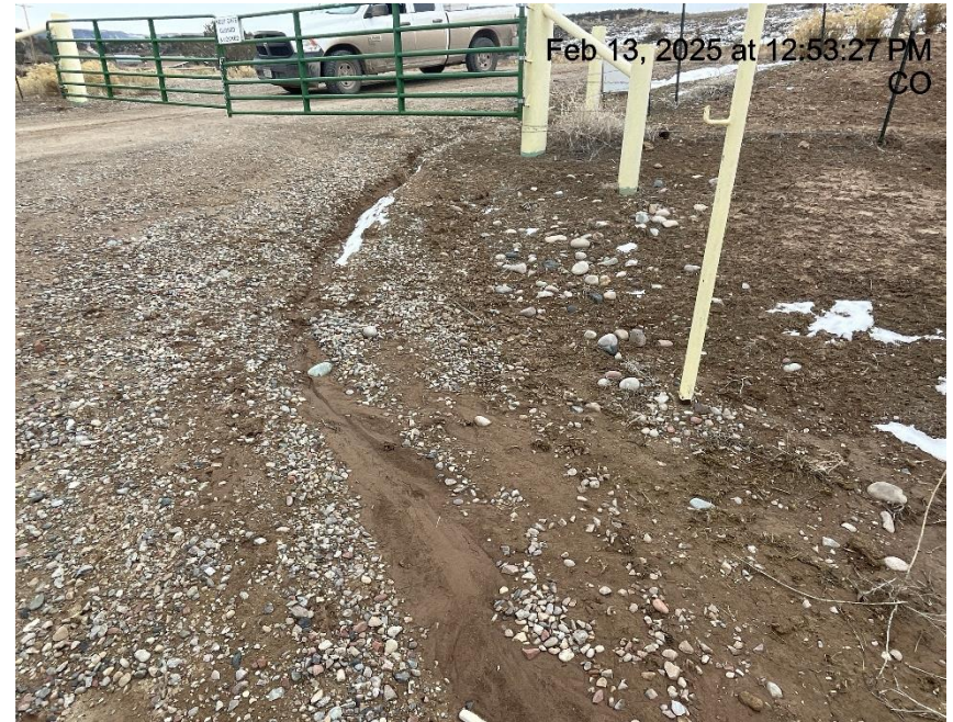
Photo # 5647 Erosion & transport of sediment/insufficient BMP's
