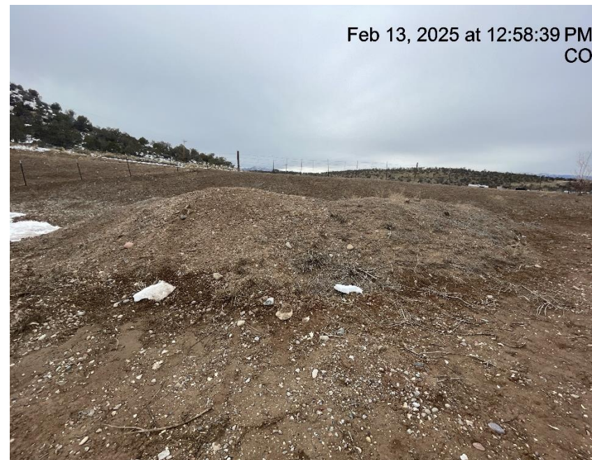
Photo # 5641 Stockpiled soils with no BMP's
