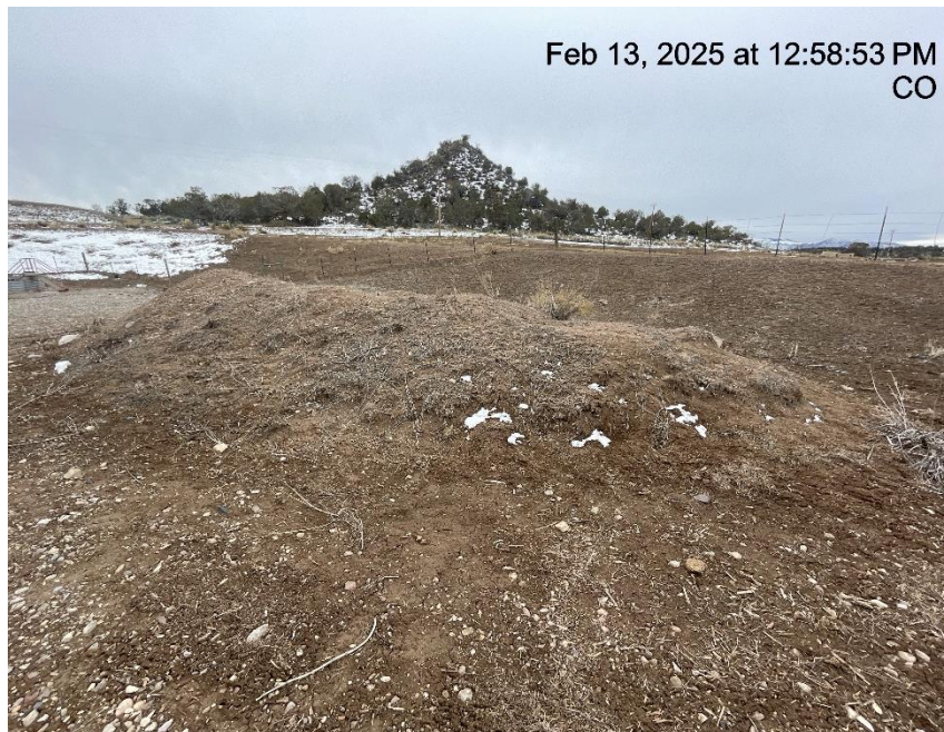
Photo # 5642 Stockpiled soils with no BMP's
