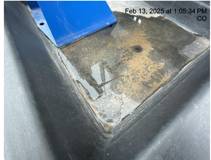
Photo # 5639 Failure to maintain chemical BMP – Chemical tank containment approximately 7/8 full of fluid/BMP insufficient to contain possible spill (additionally standing fluid starting to accumulate on top of the containment is also wildlife hazard)
