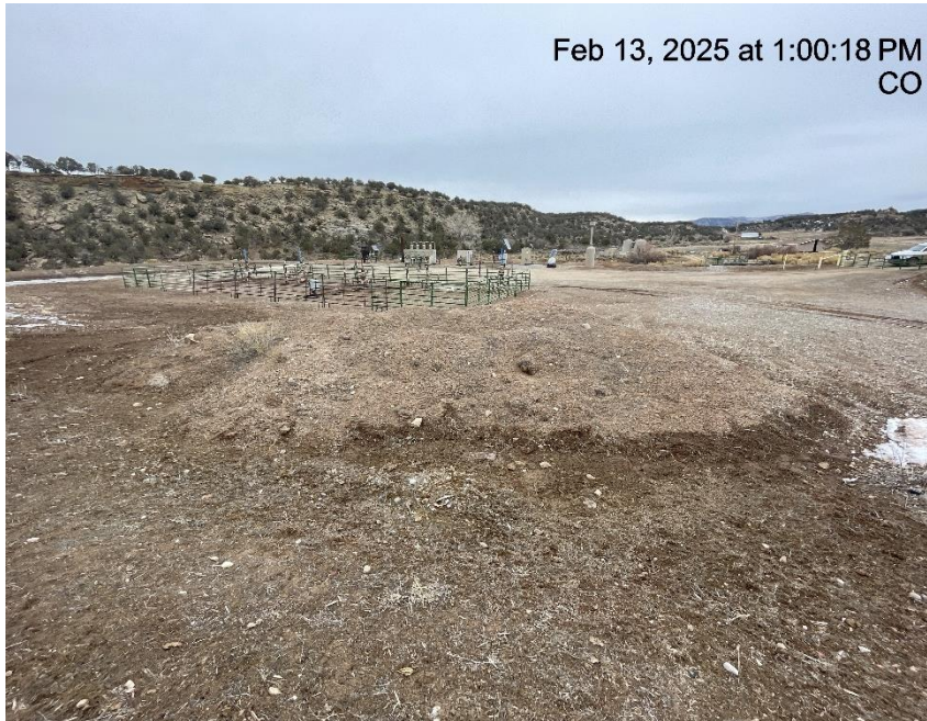
Photo # 5644 Stockpiled soils with no BMP's
