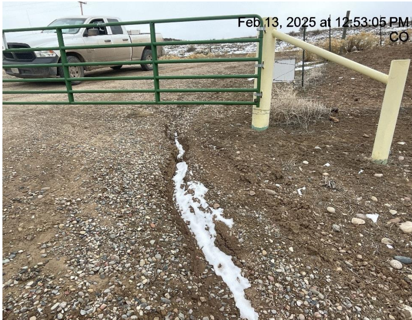
Photo # 5646 Erosion & transport of sediment/insufficient BMP's
