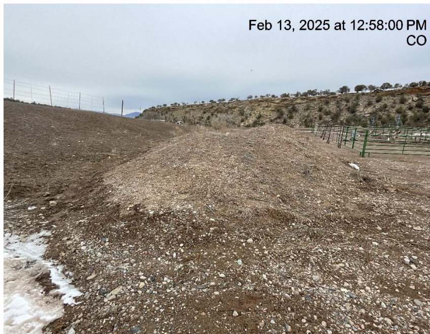
Photo # 5640 Stockpiled soils with no BMP's
