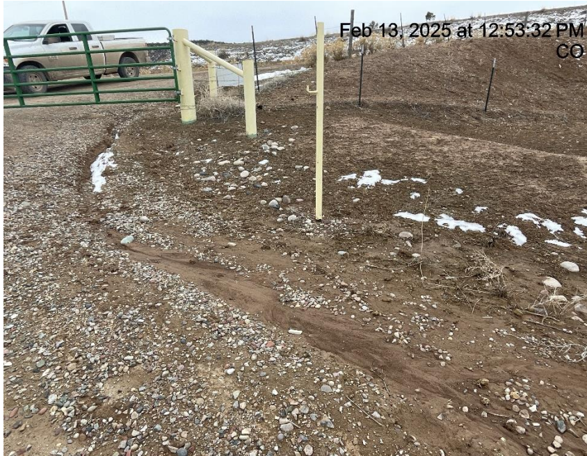
Photo # 5648 Erosion & transport of sediment/insufficient BMP's
