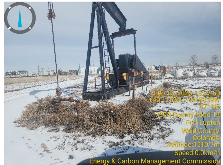
Photo 2 Dead vegetation around the wellhead.
