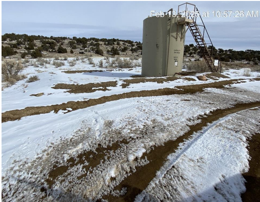
Tank berm insufficient
