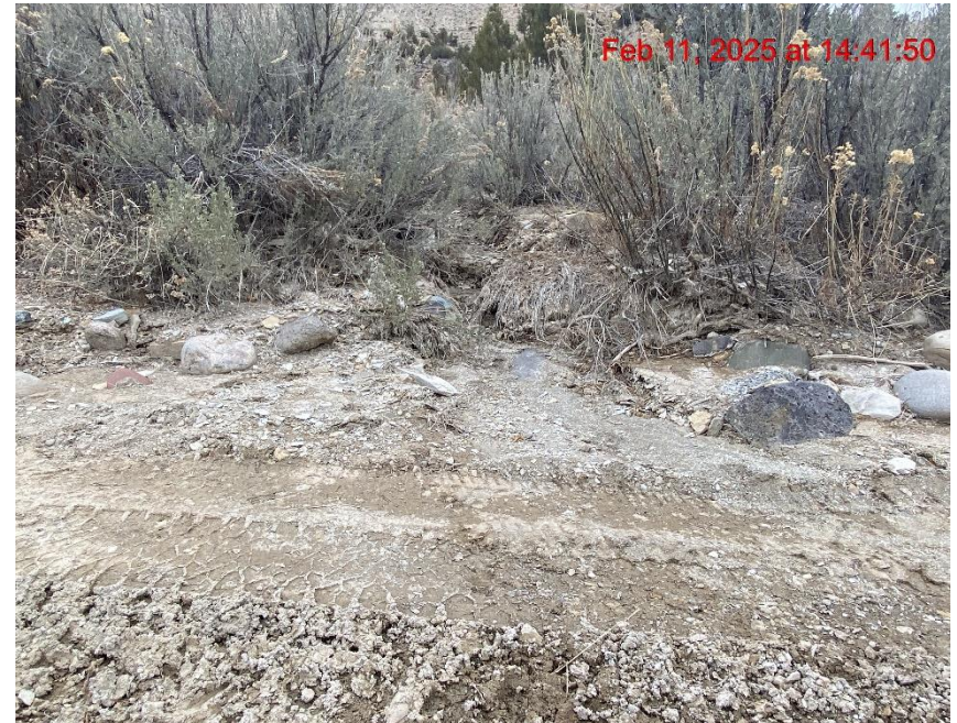
Sediment Transported onto Access Road/No BMPs – Photo #06574
