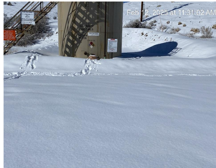
Tank berm insufficient
