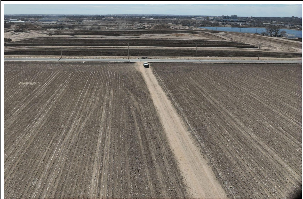
Drone Photo March 2024 - Facing South
