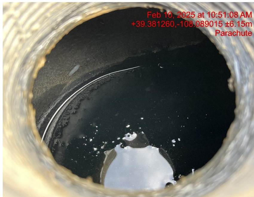
Photo # 4443 Failure to maintain chemical BMP/chemical containment approximately 3/4th full of fluid/not sufficient to contain possible spill
