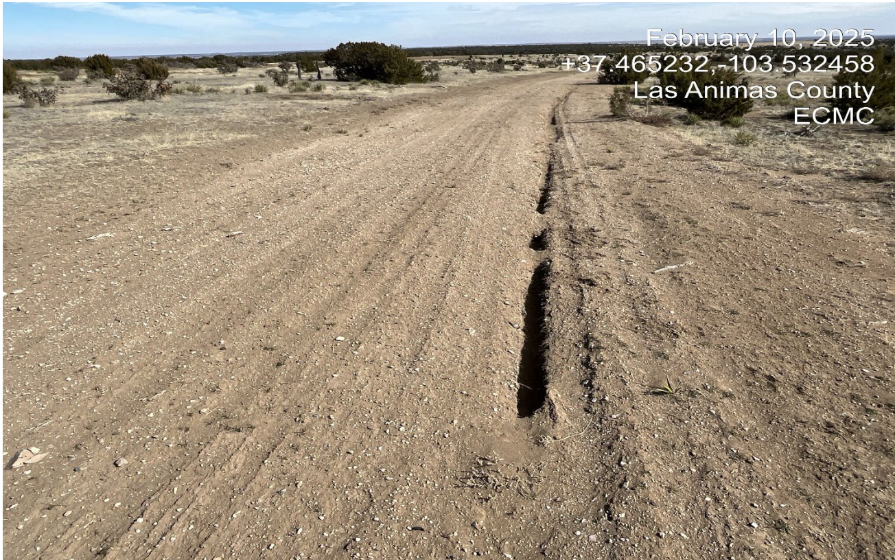
Photo 6. Facing east toward the flowline disturbance. There is subsidence along the flowline that needs to be filled in.
