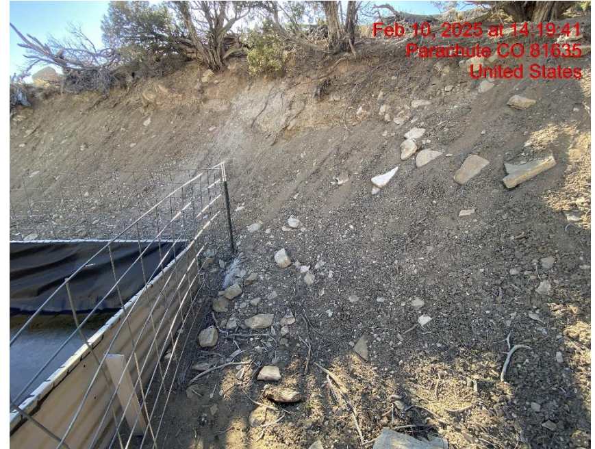
Insufficient Erosion Controls – Photo #06556
