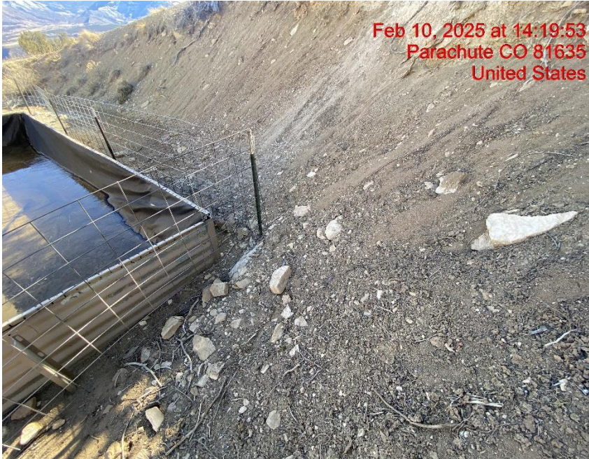
Insufficient Erosion Controls – Photo #06557
