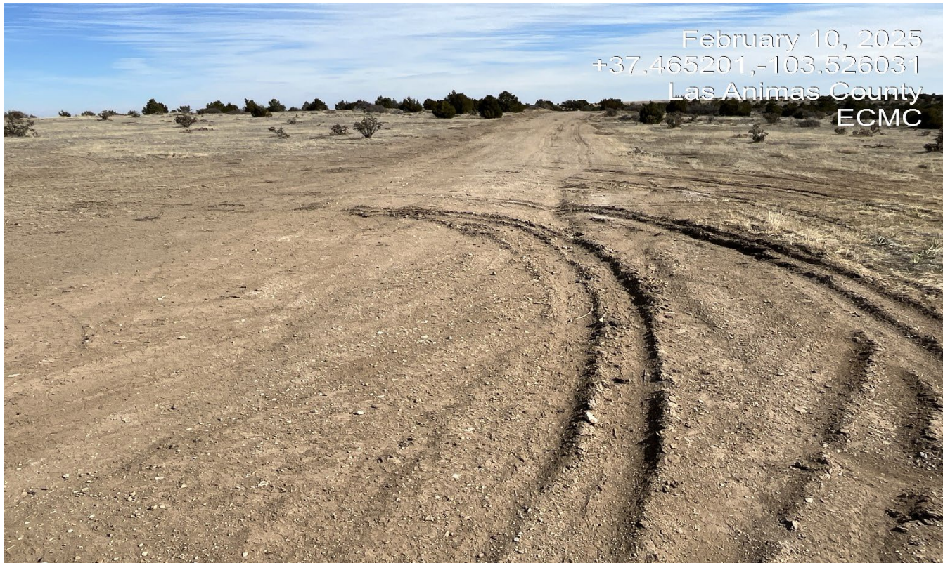
Photo 6. Facing east toward the flowline disturbance. The vegetation is not establishing along the flowline and there are vehicle tracks which are causing unnecessary disturbance. The flowline must be reclaimed and stabilized.
