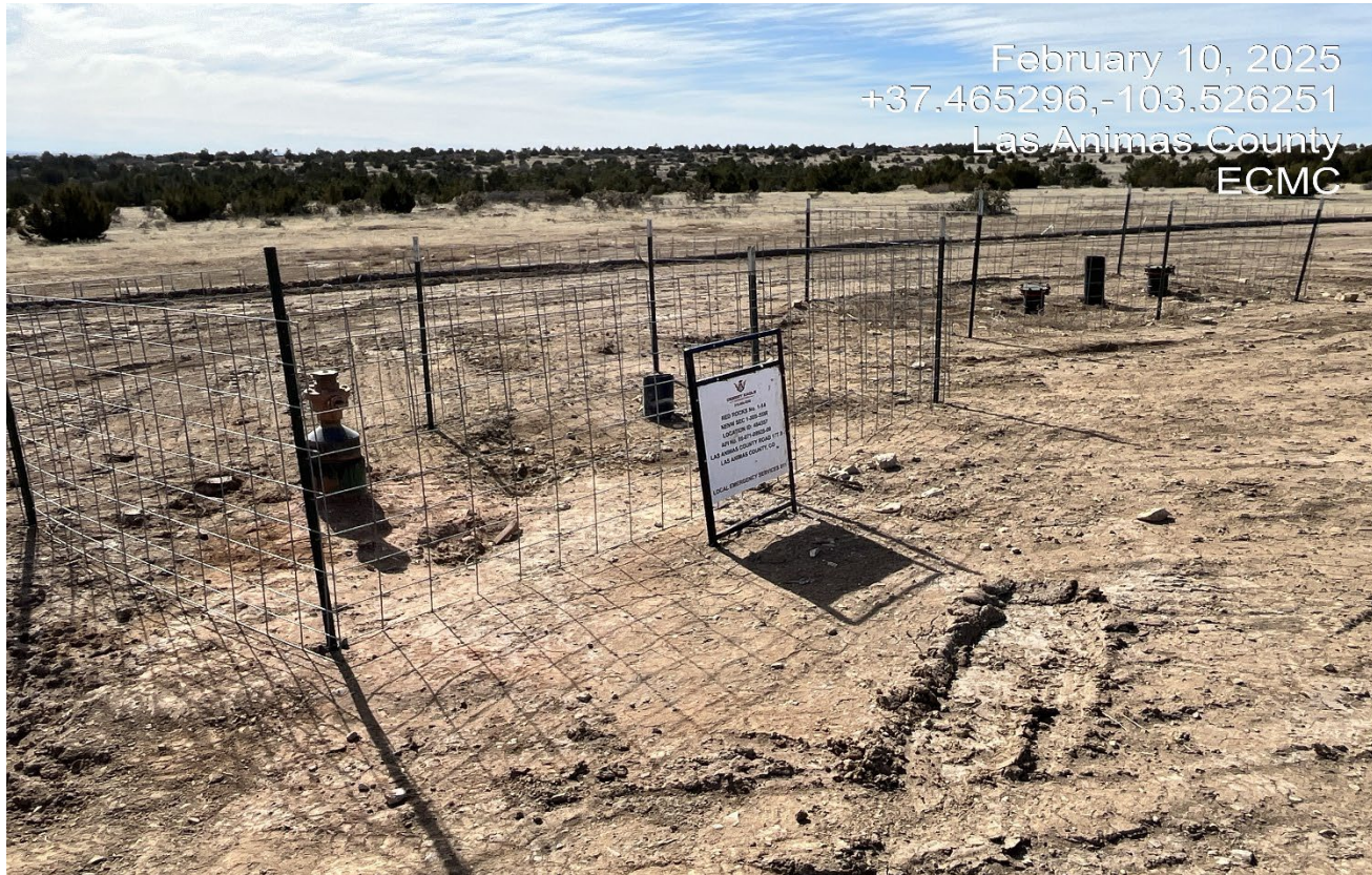
Photo 4. Facing at the wellhead. There is red drill cutting still present at the wellhead. Sign and fences have been reinstalled.
