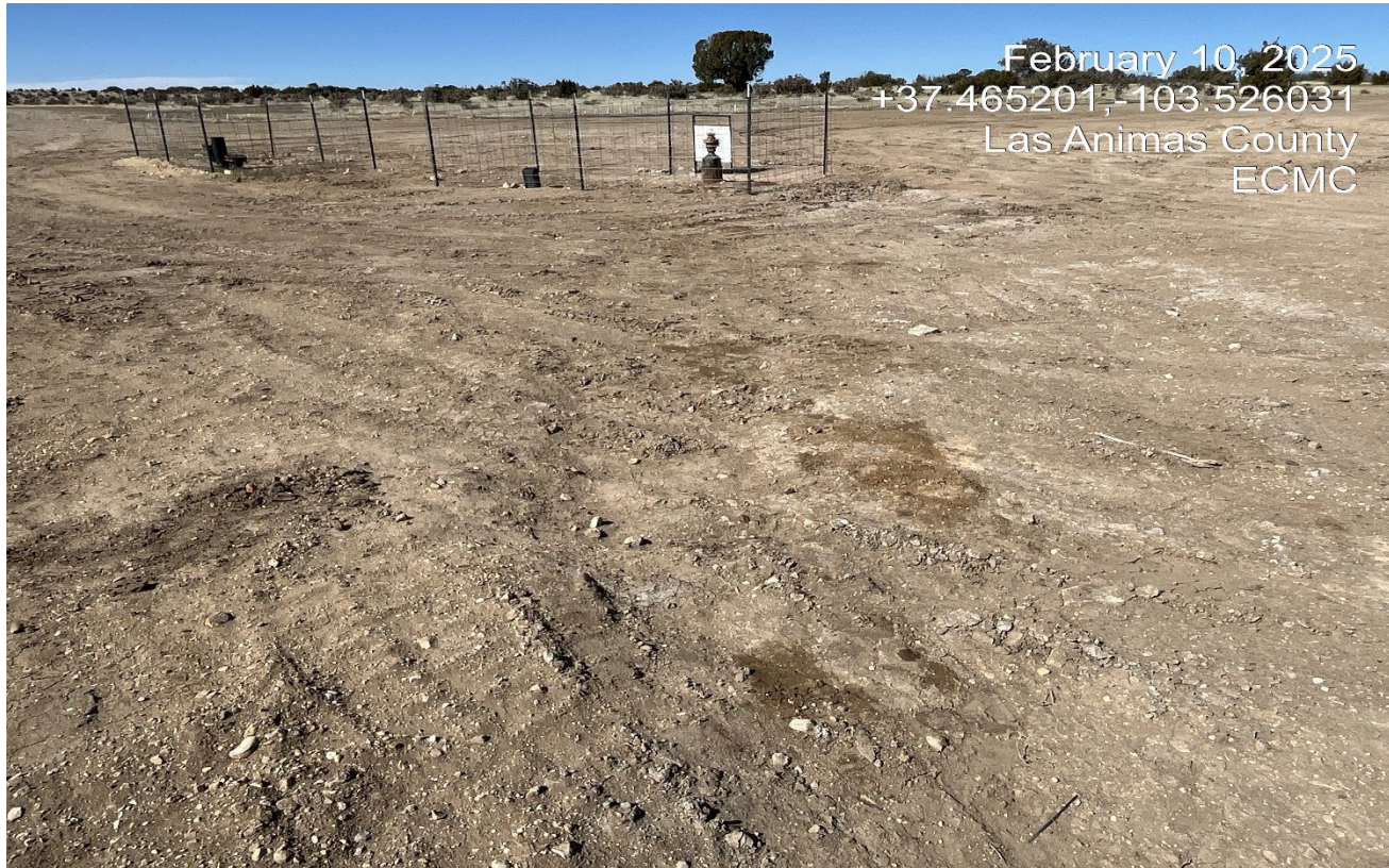
Photo 5. Facing northwest at the location. There are stained soils southeast of the wellhead that have not been cleaned up. Previous CA was not completed.
