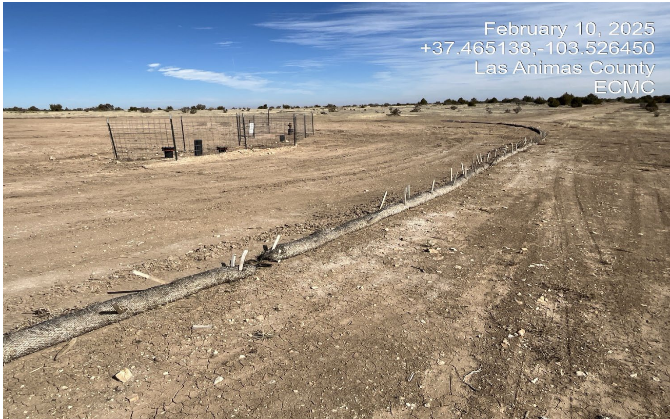
Photo 7. Facing northeast at the location. The wattles have been reinstalled at the south side of the location. Disturbed areas will need to be reseeded.
