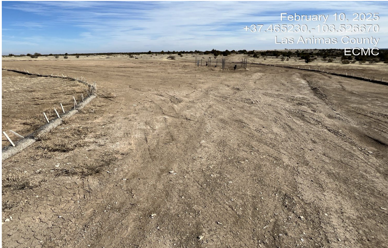
Photo 8. Facing northeast at the location. The wattles have been reinstalled at the south side of the location. Disturbed areas will need to be reseeded. Compacted soils must be decompacted by cross ripping to at least 8 inches.
