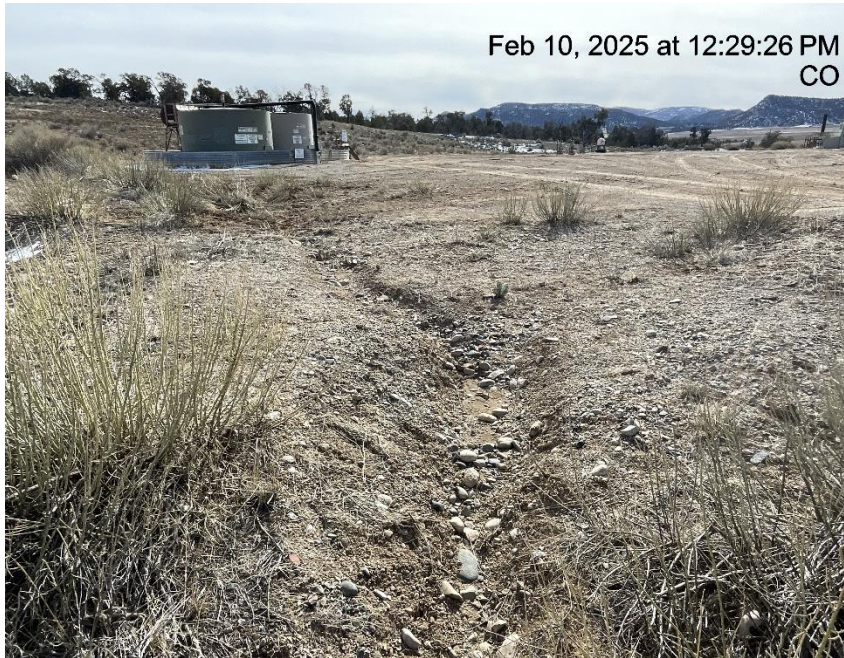
Photo # 4647 Erosion & transport of sediment off location /insufficient BMP's
