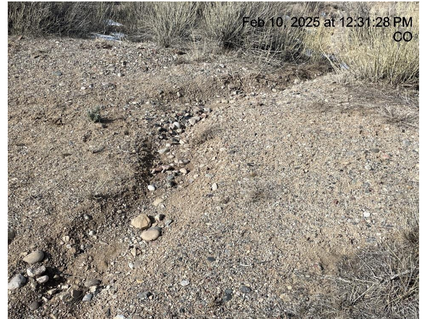
Photo # 4648 Erosion & transport of sediment off location /insufficient BMP's
