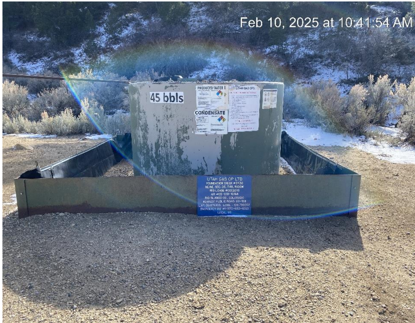
Tank berm inadequate
