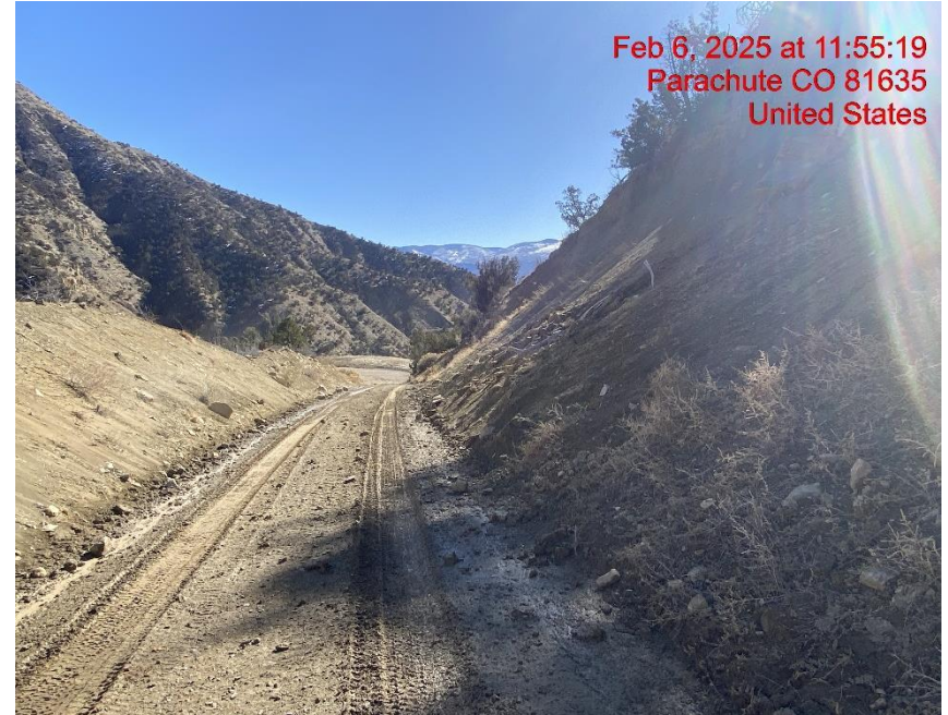
Cut Slope Eroding onto Access Road – Photo #06509
