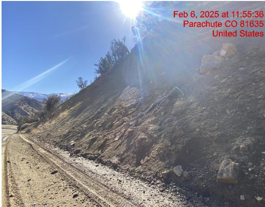
Cut Slope Eroding onto Access Road – Photo #06510
