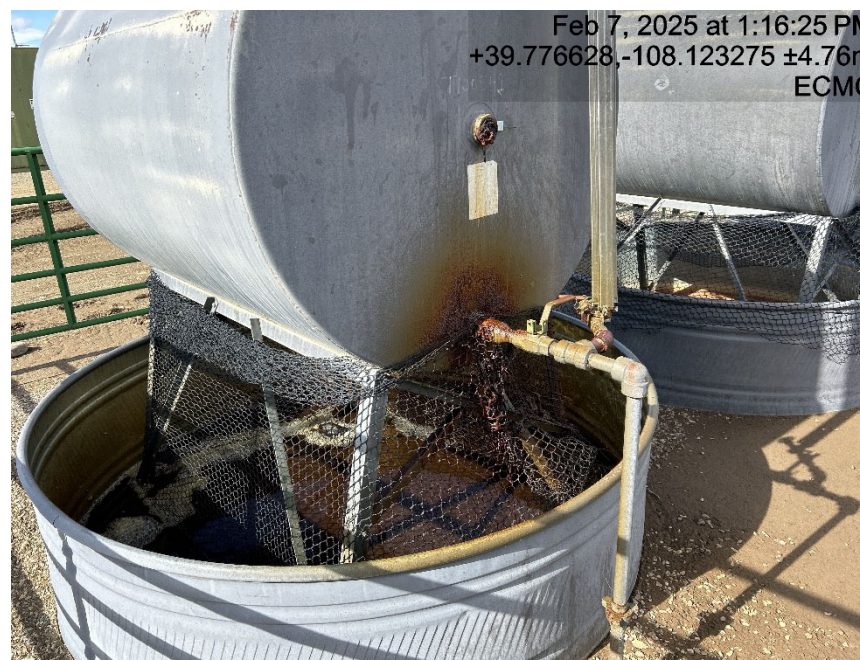
Tank leaking
