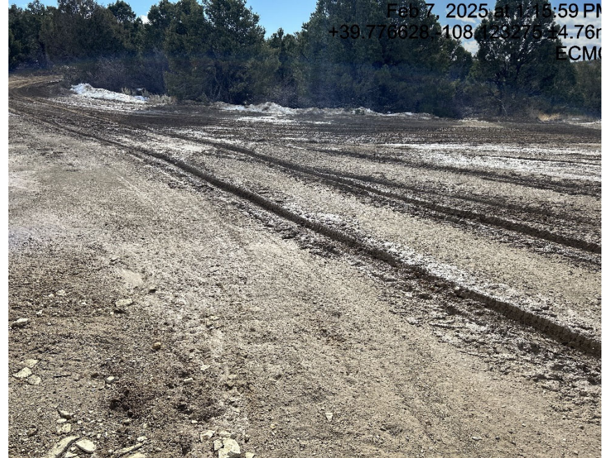
Lack of stabilization/compaction
