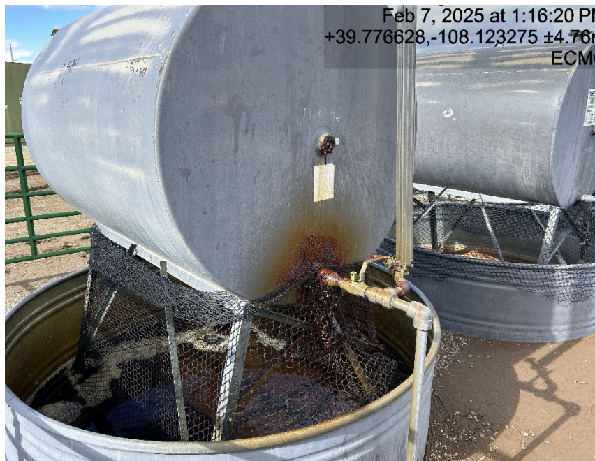
Tank leaking
