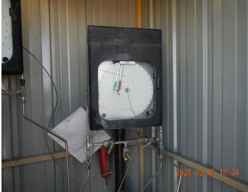
5. Gas meter inside meter shed.
