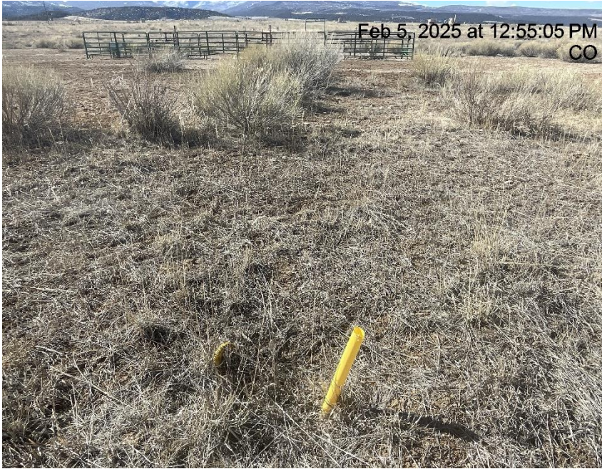
Photo # 3687 Improperly marked deadman
