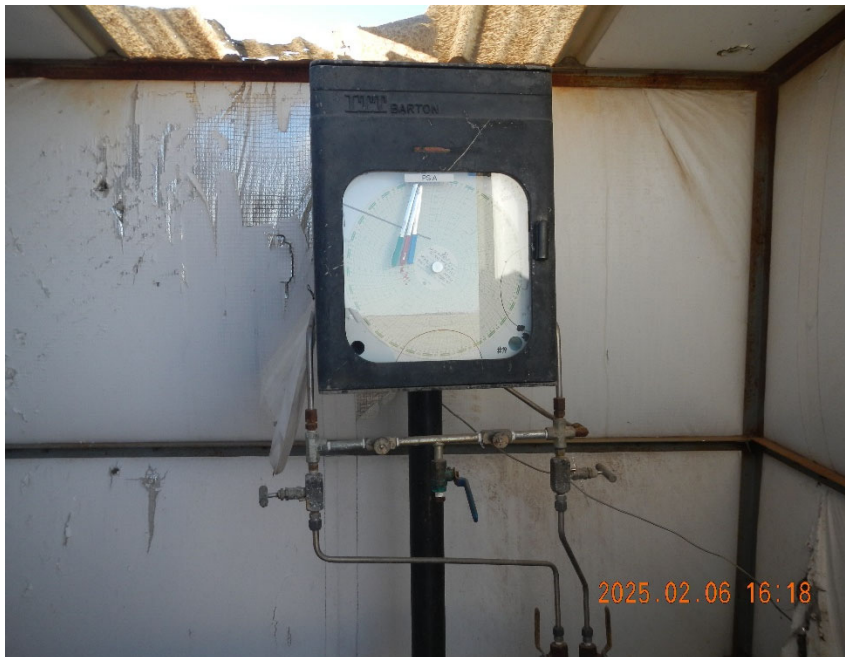
7. Gas meter inside meter shed. Note roof damage at top of frame.
