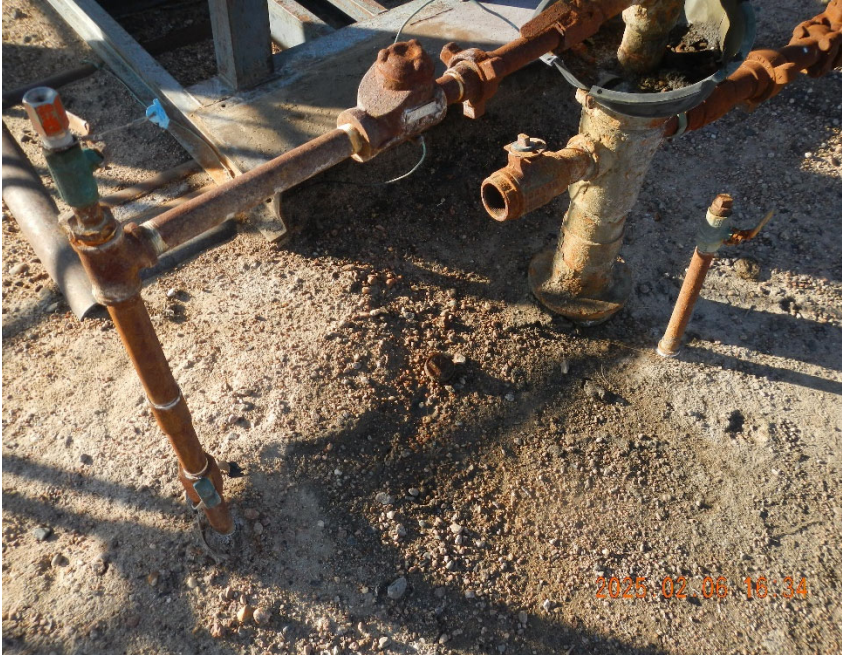
3. View of release location at wellhead. Note absence of fine sand at release point.
