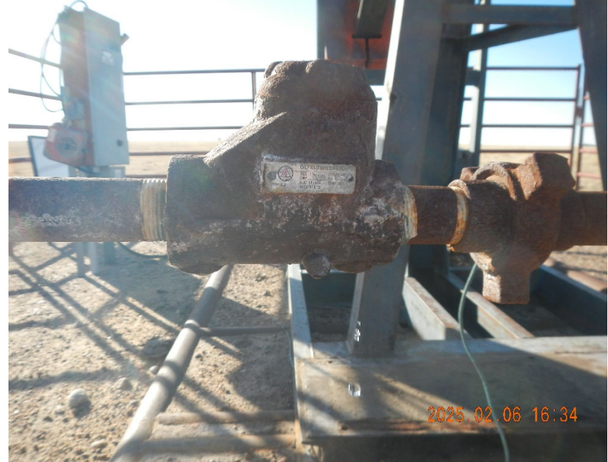
4. View of leaking check valve. Note salt staining on check valve body.
