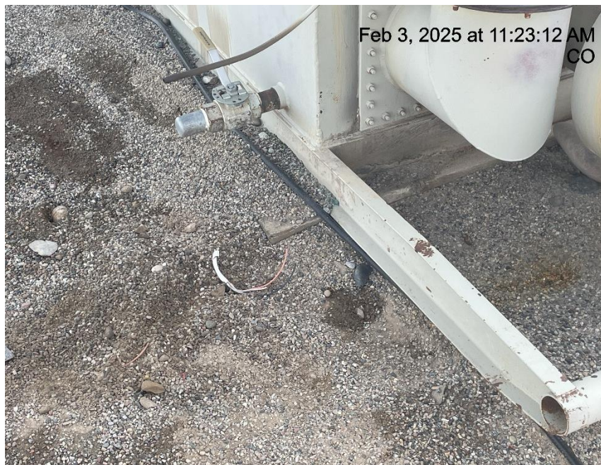
Photo # 3009 Staining near separator
