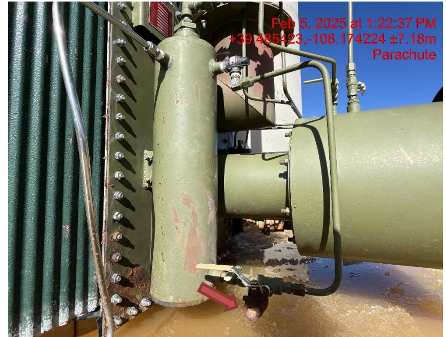
Photo # 4211 PRV vent line on tank heater does not comply with CECMC pressure safety device rules
