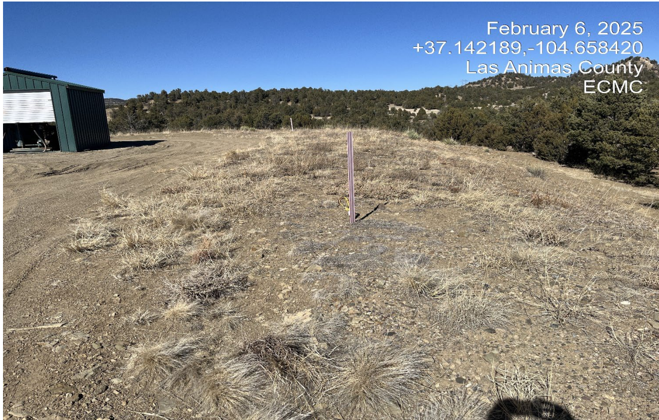
Photo 3. Facing north along the fill slope which is stabilized with vegetation.
