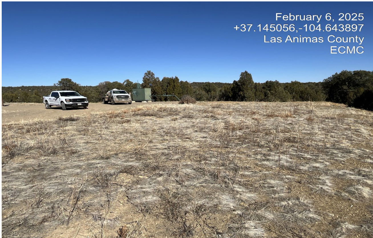
Photo 2. Facing east along the fill slope which is stabilized with vegetation.
