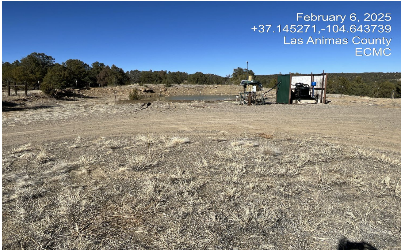
Photo 1. Facing north at the location. The water level was above freeboard.
