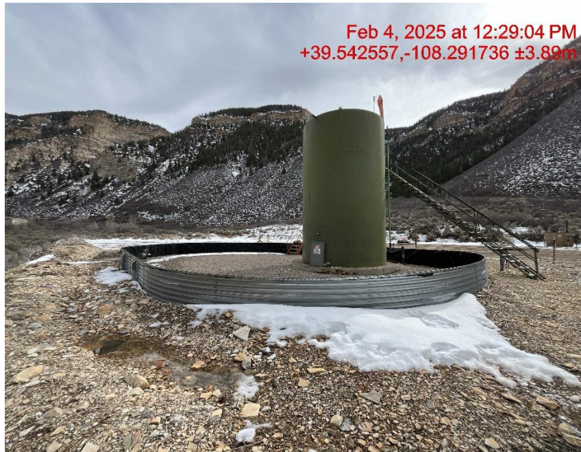
Photo # 4064 NW corner of location
