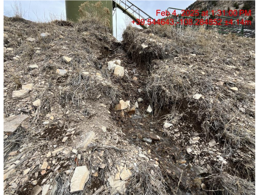
Photo # 4119 Failure to minimize erosion & transport of sediment off location/insufficient BMP's
