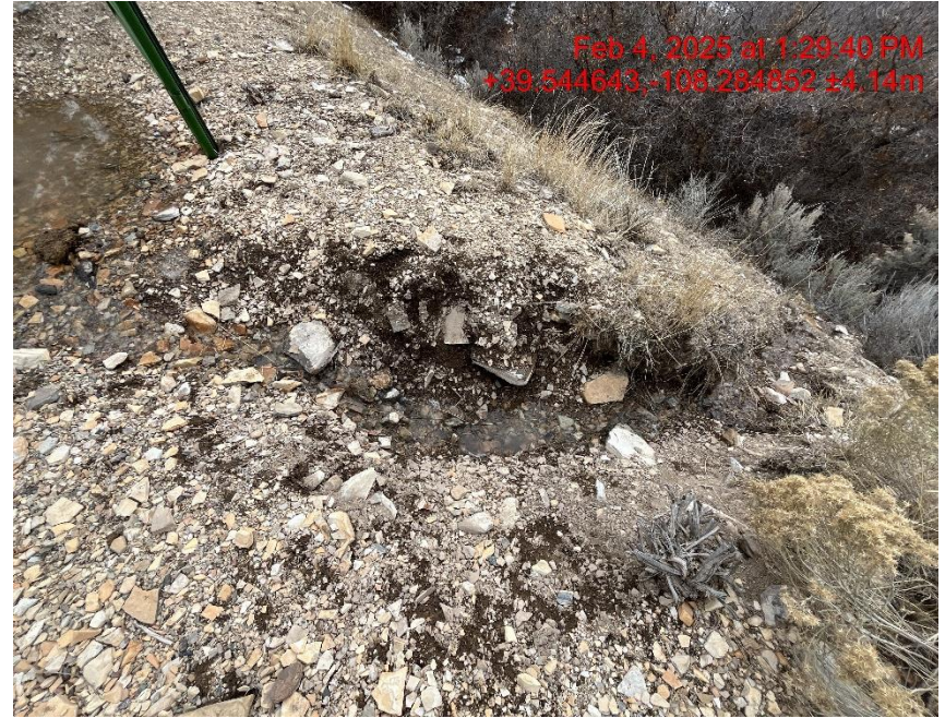
Photo # 4115 Failure to minimize erosion & transport of sediment off location/insufficient BMP's
