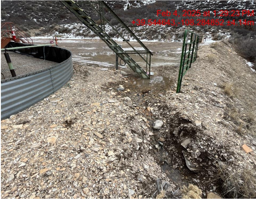
Photo # 4114 Failure to minimize erosion & transport of sediment off location/insufficient BMP's
