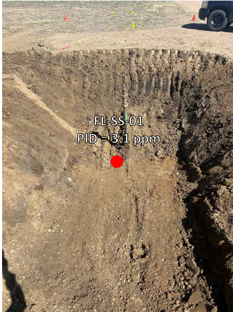
Looking east at flowline Pt A
