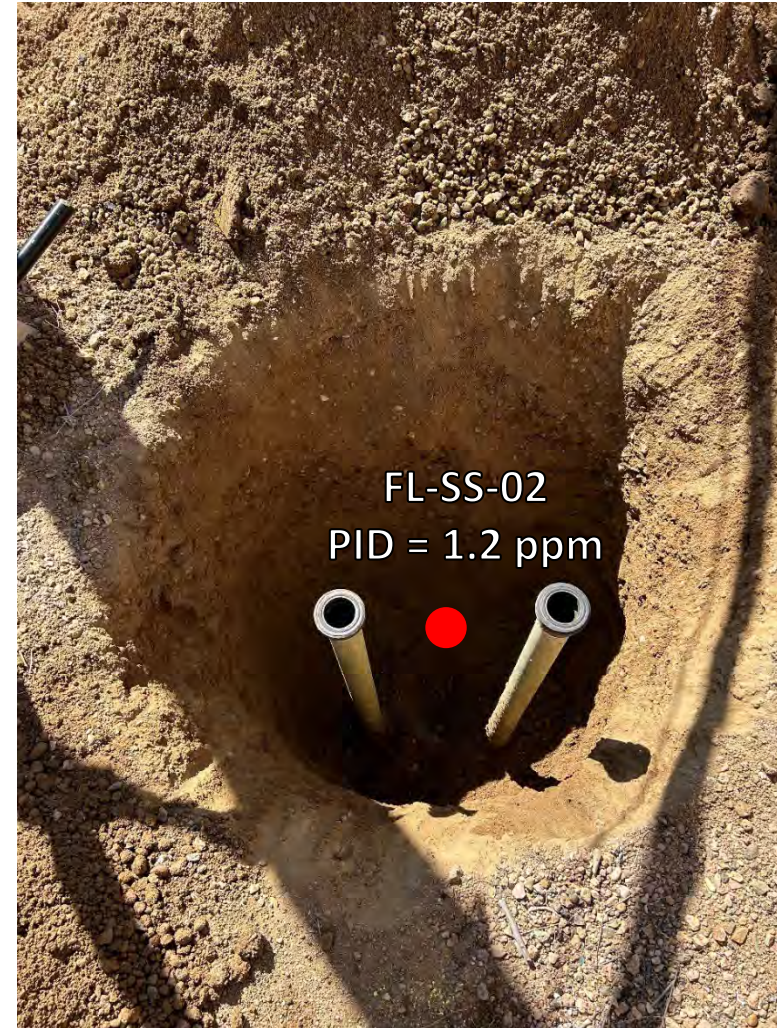
Looking west at flowline Pt B/terminus at separator
